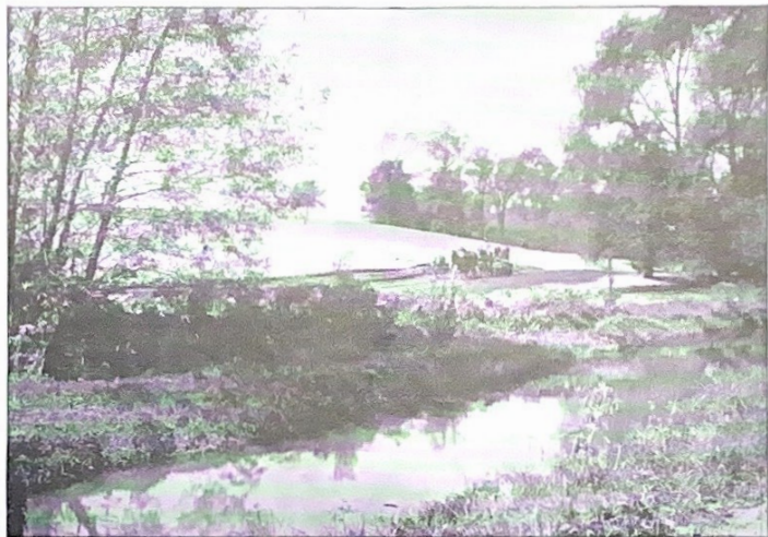
Work proceeding on line of Cameron Parkway, along Spring Creek.—1906
